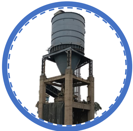
Fly ash silo – 420M3 Dense phase pneumatic handling system
