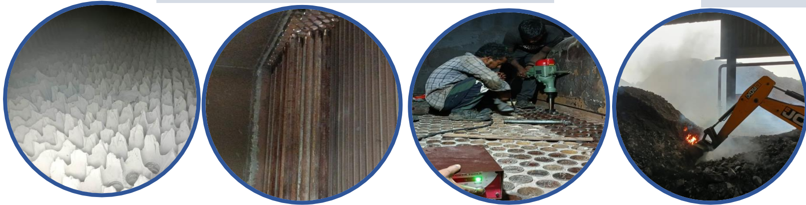
APH Tubes fouling /Replacement in Oct'21
